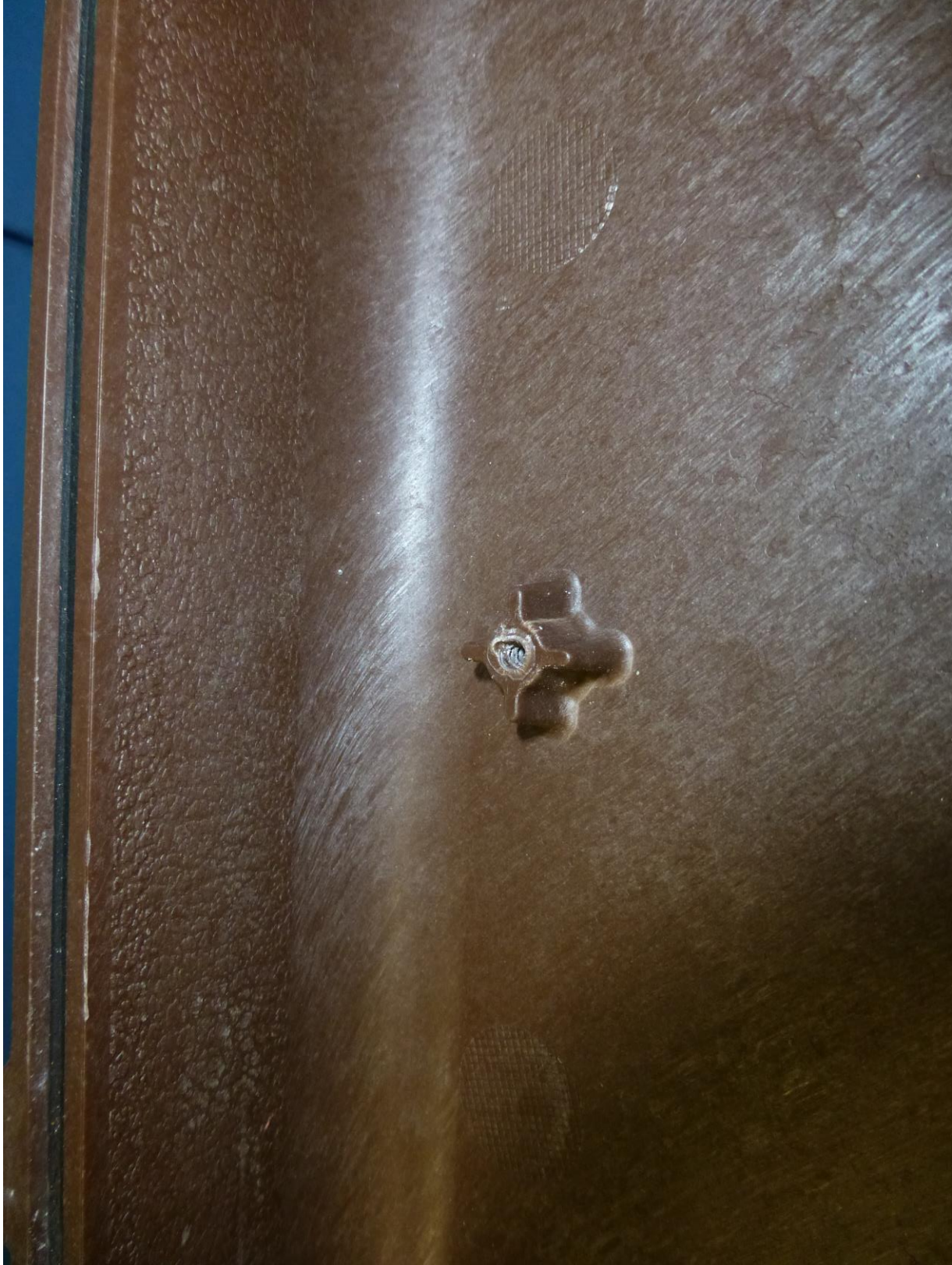
Photograph 38 Impact with Mass – Post Inspection - Typical
